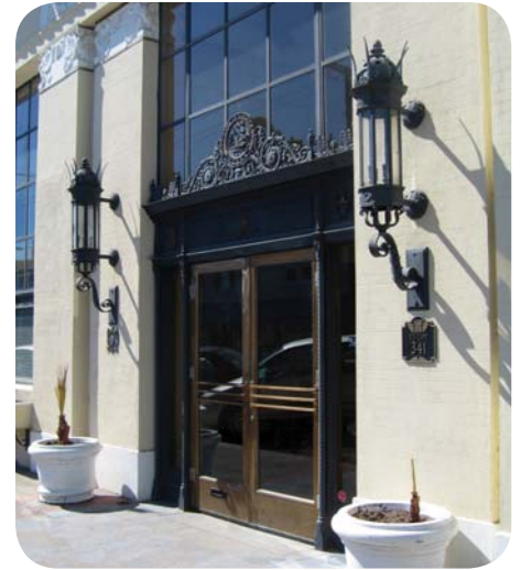
Figure 5.9.3 These wall mounted lights provide sufficient light to ensure freestanding fixtures are unnecessary.
