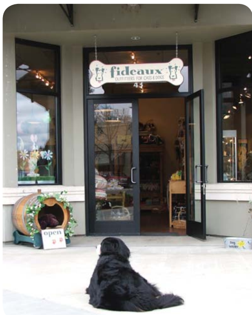
Figure 5.7.1 The storefront is the most important architectural feature of many commercial buildings.
