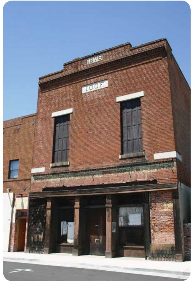
Surface cleaning should be undertaken with the gentlest means possible. Sandblasting and other harsh cleaning methods that may damage historic building materials is not allowed
