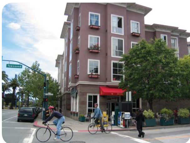
Figure 5.3.1 Buildings should be placed along the front setback to provide the desired pedestrian environment.
