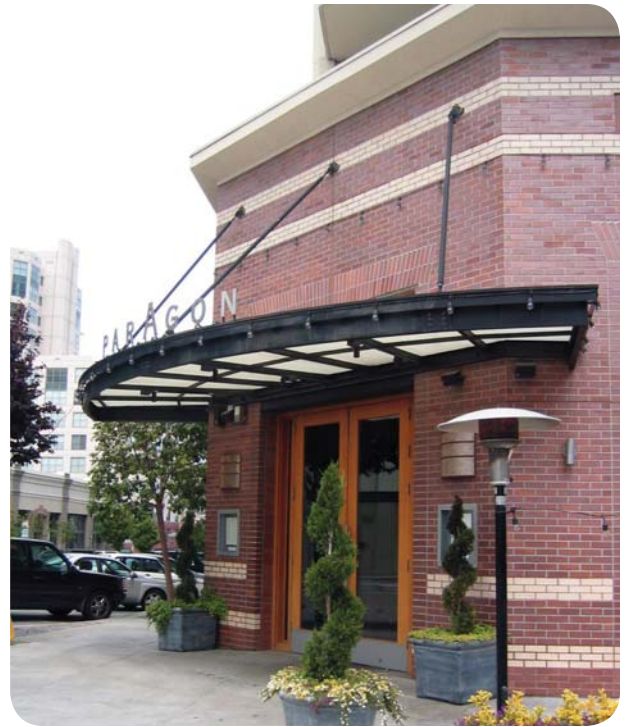
Figure 5.4.21 Accent brick banding is a relatively simple design technique to create interest in the facade.
