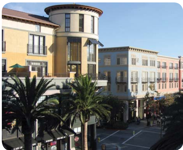
Figure 5.4.15 This building height is appropriate for a mixed-use infill project and incorporates an attractive corner element.
