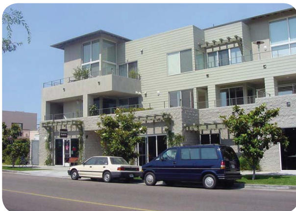
Figure 5.4.8 a-c Balconies on upper floors should be designed with special care and attention to detail to ensure that they add to rather than detract from the building.
