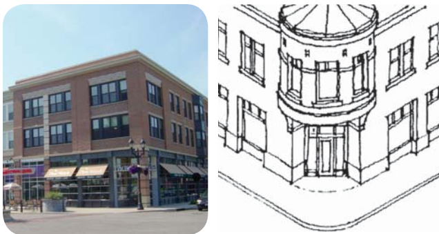
Figure 5.4.5 a-b Facade treatments at intersections should be holistic and continue on all sides of the buildings visible from the street.
