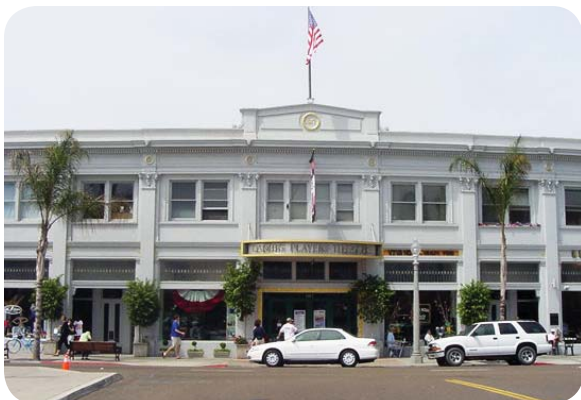
Figure 5.4.6 Windows on upper floors should be compatible with windows and openings on the first floor.
